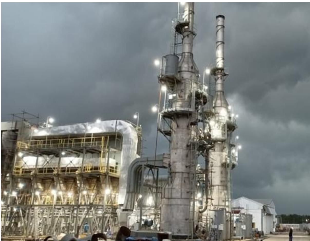
(India's first FGD in Battery Breaking unit at Haldia, West Bengal.)
